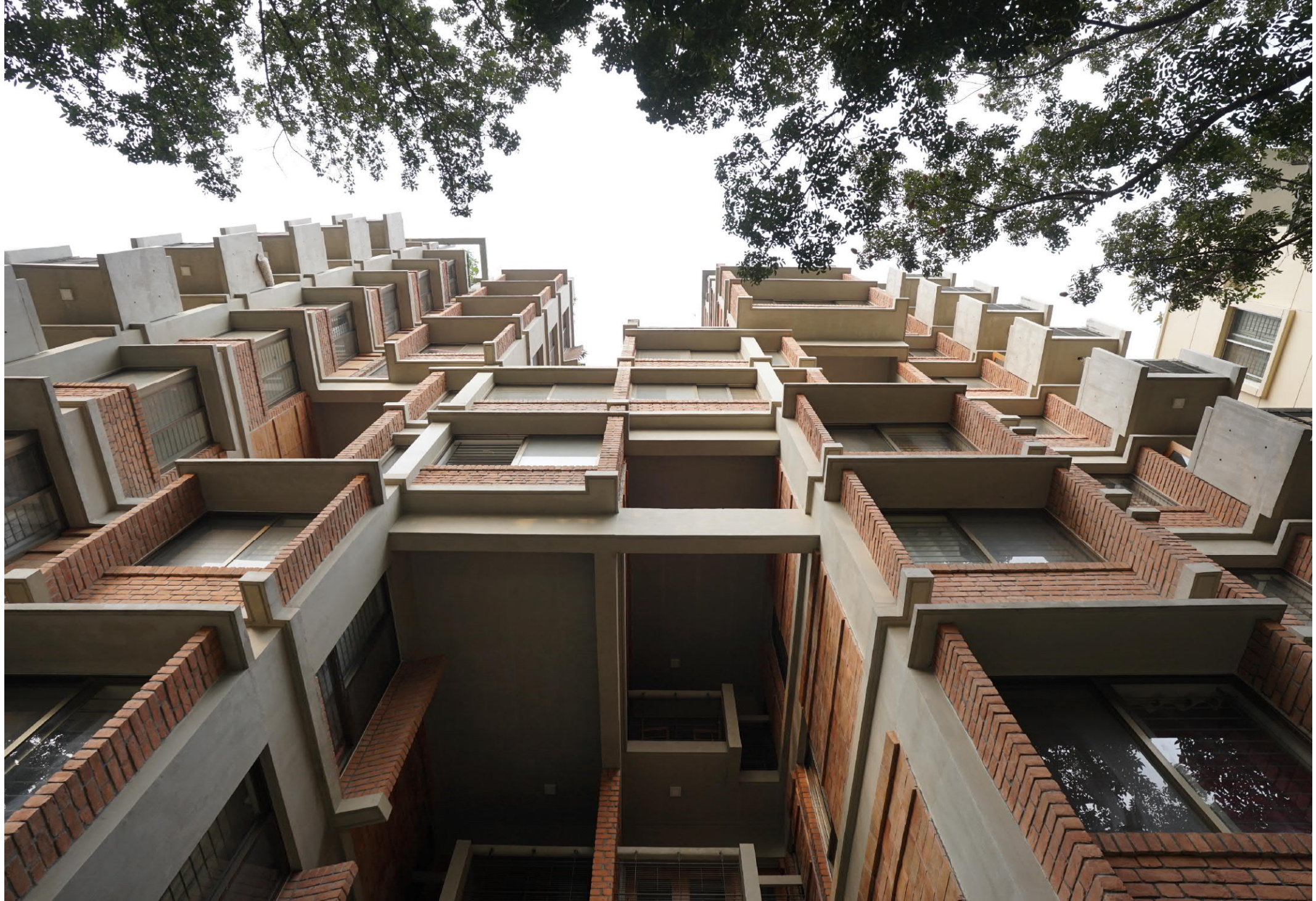
AAKASH APARTMENT TOWER
